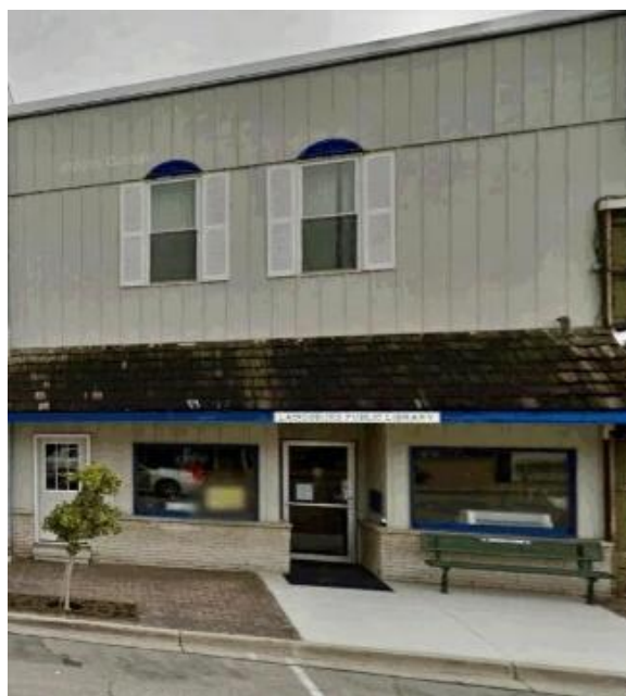
A front view of the Laingsburg Public Library is seen here.
